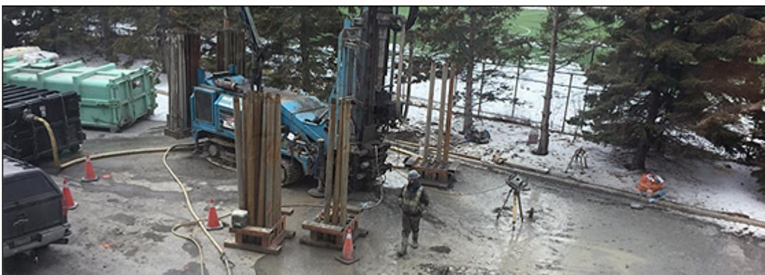
The drilling for the geothermal system began in mid-April. This was completed by mid-May, with excavation completed in June. For a full story on the ground source exchange system for the OAA HQ, [click here](#).
