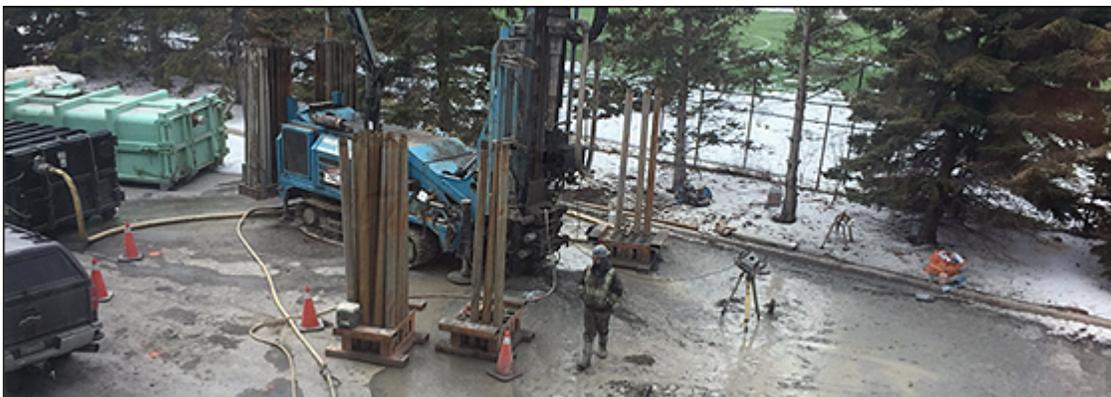
The drilling for the geothermal system began in mid-April. This was completed by mid-May, with excavation completed in June. For a full story on the ground source exchange system for the OAA HQ, [click here](#).
